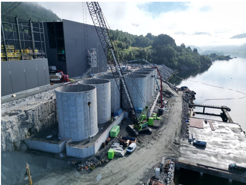
Picture 2: Installed prefabricated concrete elements for product silos.
